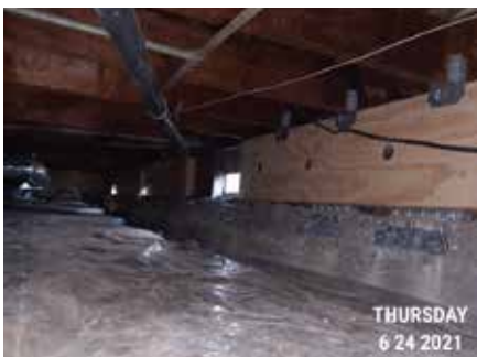
CRAWL SPACE POST-RETROFIT #2
