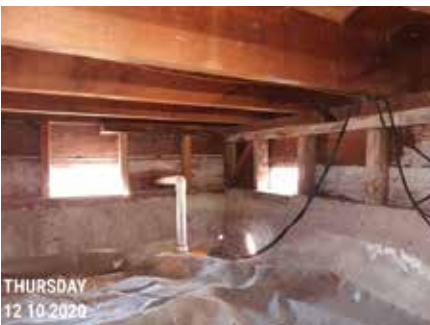
CRAWL SPACE PRE-RETROFIT #1
