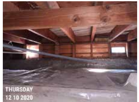
CRAWL SPACE PRE-RETROFIT #3
