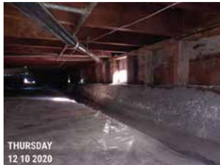
CRAWL SPACE PRE-RETROFIT #2
