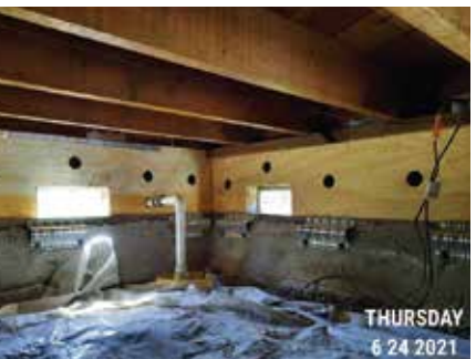
CRAWL SPACE POST-RETROFIT #1
