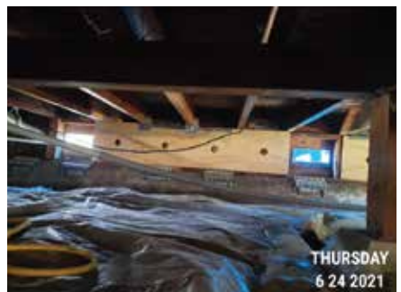
CRAWL SPACE POST-RETROFIT #3
