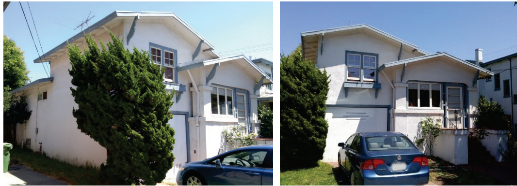
Figure C.1.5-2 Split level configuration in a living-space-over-garage dwelling.
