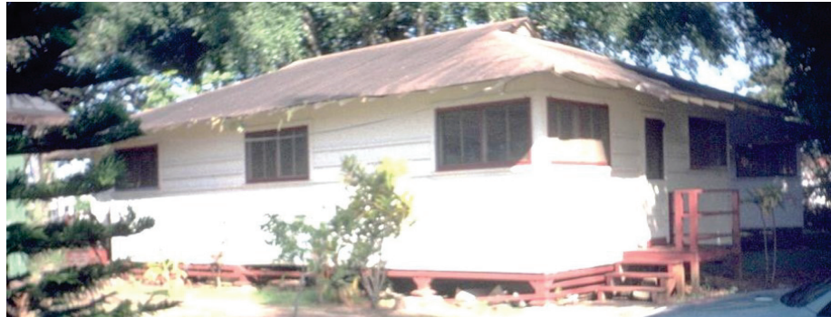
Figure C.8.1-2 Dwelling on post and pier foundation.
