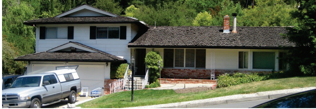
Figure C.1.5-1 Split level configuration in a living-space-over-garage dwelling.
