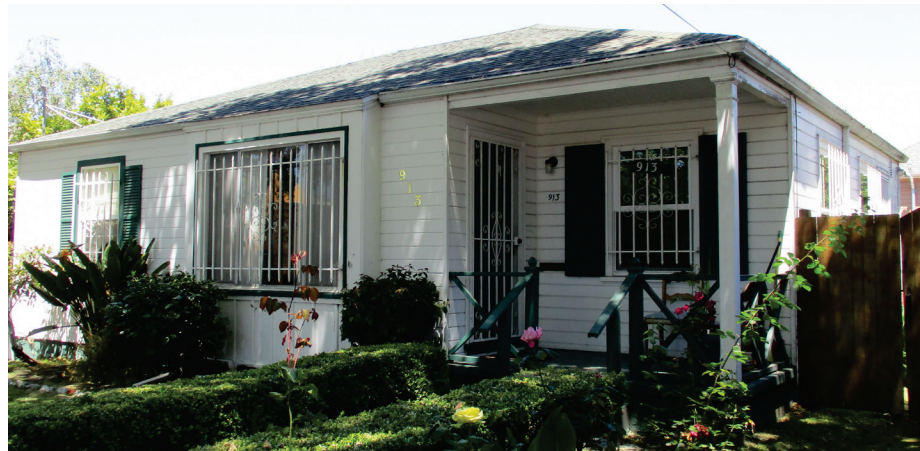
Figure C.8.1-1 Dwelling with a front porch that is set into the main dwelling footprint.
